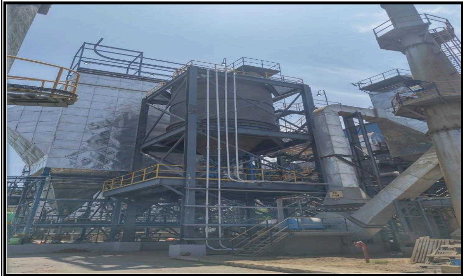
Silo installed for fly ash storage and dusting free truck loading
